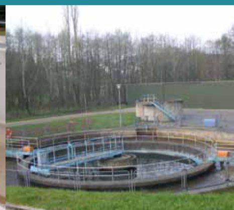
Station d'épuration, Redange
